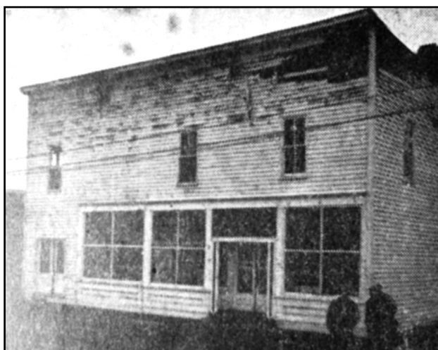
FIRE! - (December 4, 1963) - The blaze spread from the Wilson H. Smith Sales Company building to the frame building next door, owned by Halterman's Hardware, and completely gutted it before it was brought under control. The above photo does not show the side of the building into which the fire spread. The restored building now houses South Side Depot on South Main Street.
